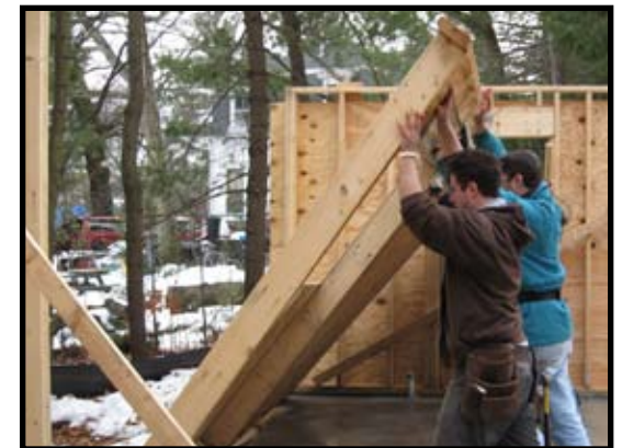
Volunteers raise the walls in Newton
